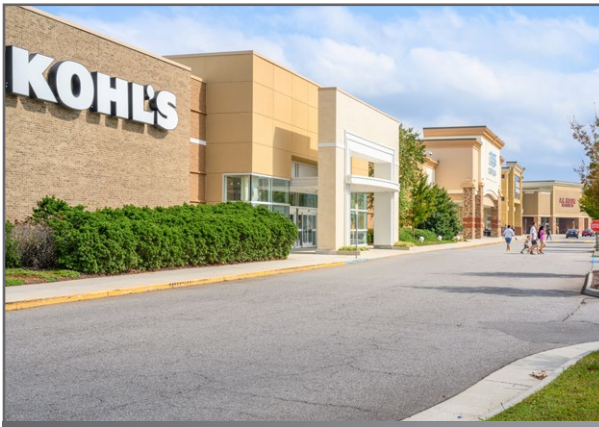
Landstown Commons, Virginia Beach, VA
